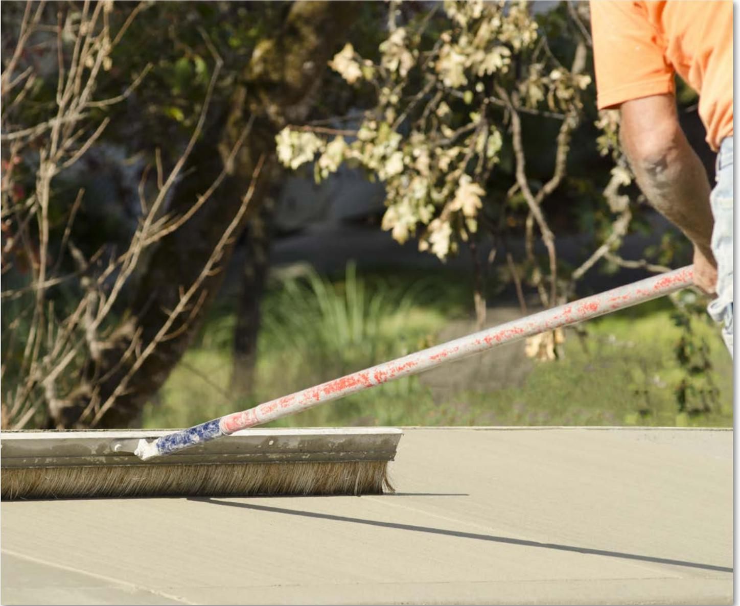
Contractor broom finishing a concrete sidewalk/curb
