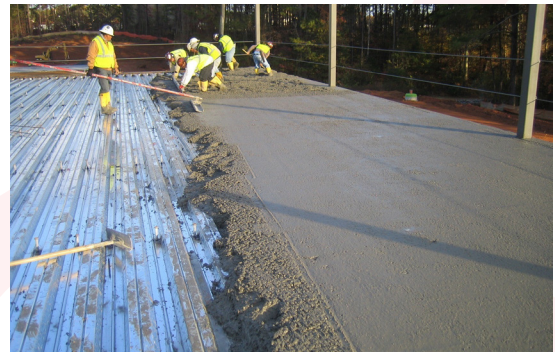
Composite Steel Deck
